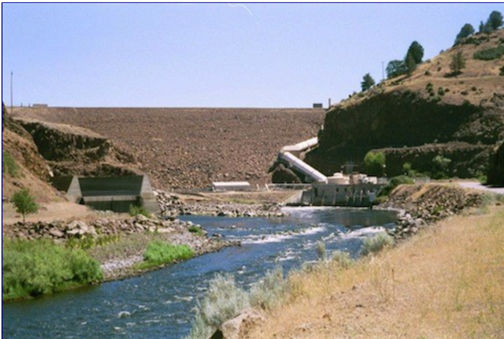
Iron Gate – most downriver of five Klamath River Dams owned and operated by PacifiCorp.
